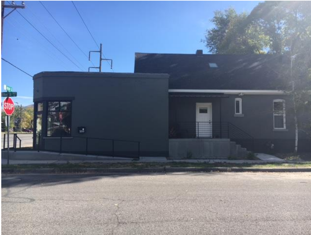
View of Western Portion of Subject Property (facing Blair Street)
